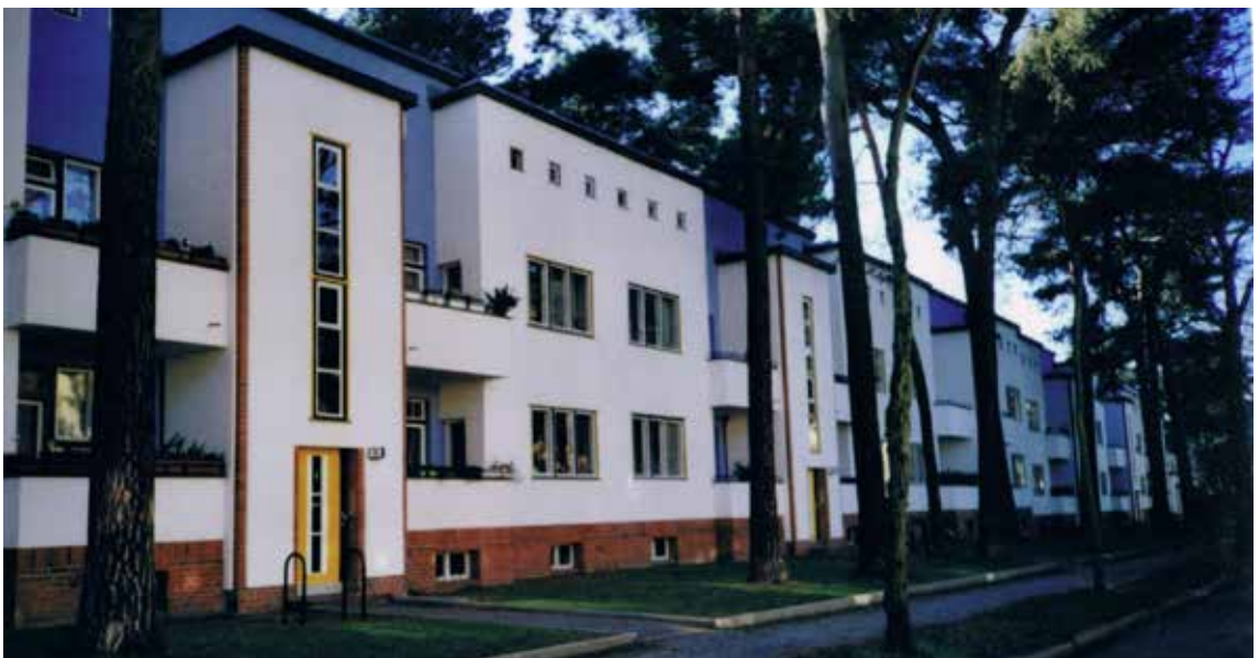
Housing project in Berlin, Germany © Wikipedia/Gyxyz
