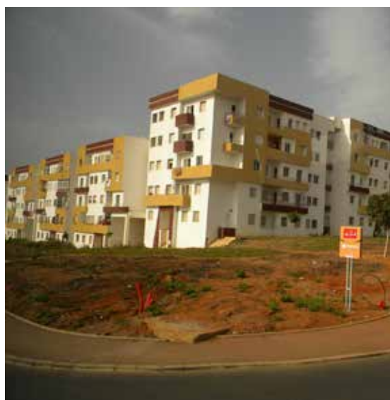
Housing units in Rabat, Morocco © UN-Habitat
